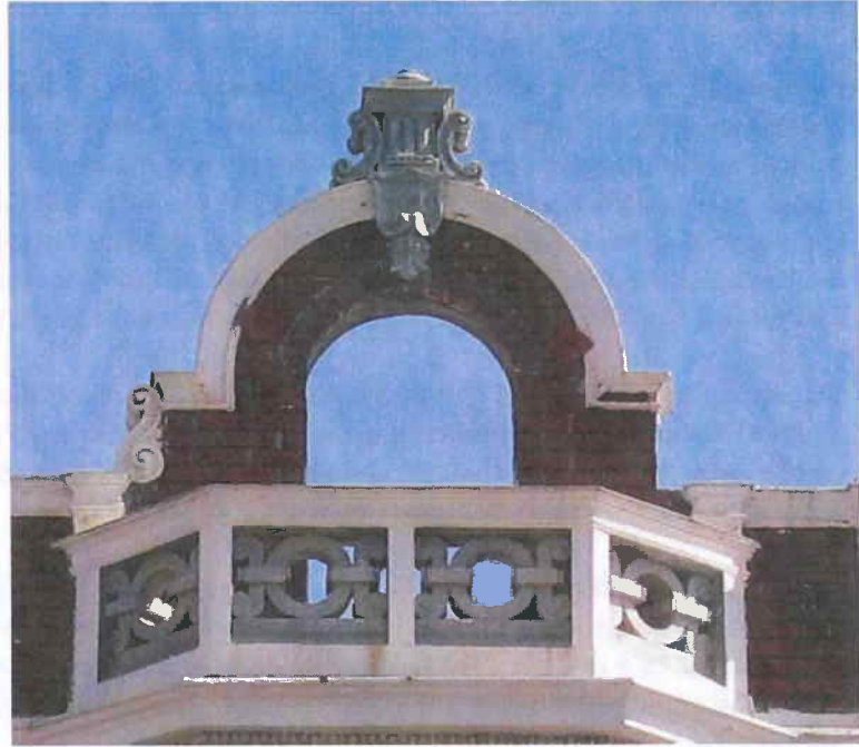
Figure 28 - 1693 Market St, parapet detail
