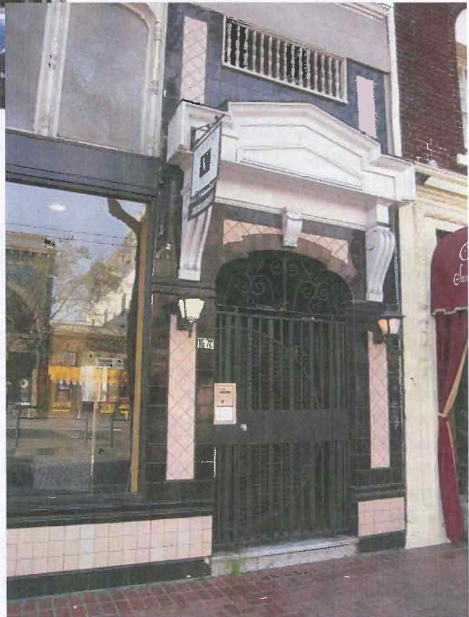
Figure 22 - 1670 Market Street entry detail
