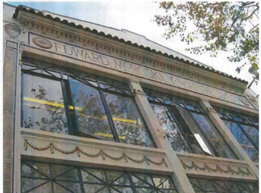
Figure 24 - 1687 Market, upper floor detail
