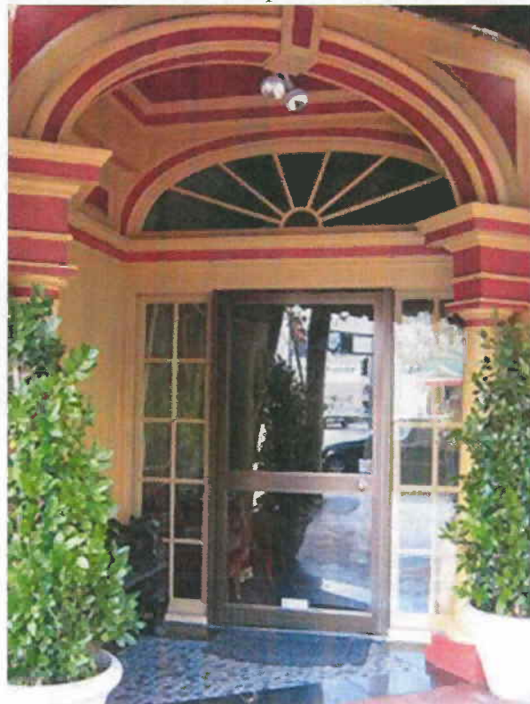
Figure 17 - 1666 Market Street, entry detail
