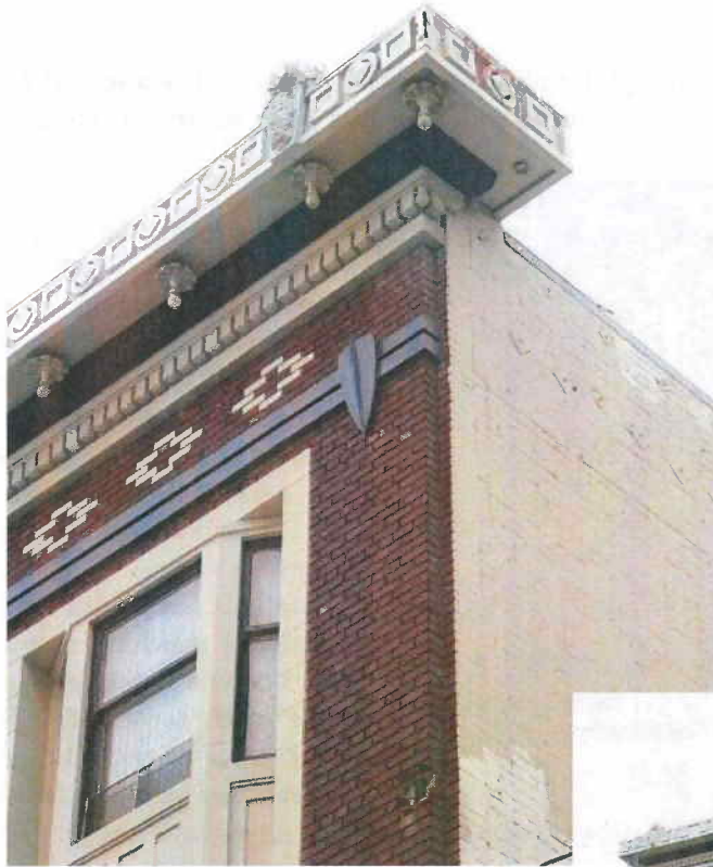
Figure 3 - 150 Franklin entablature detail
